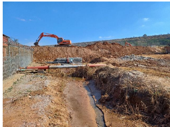
Figure 6 – One of the connection points of the new pipeline to the existing TSF.
